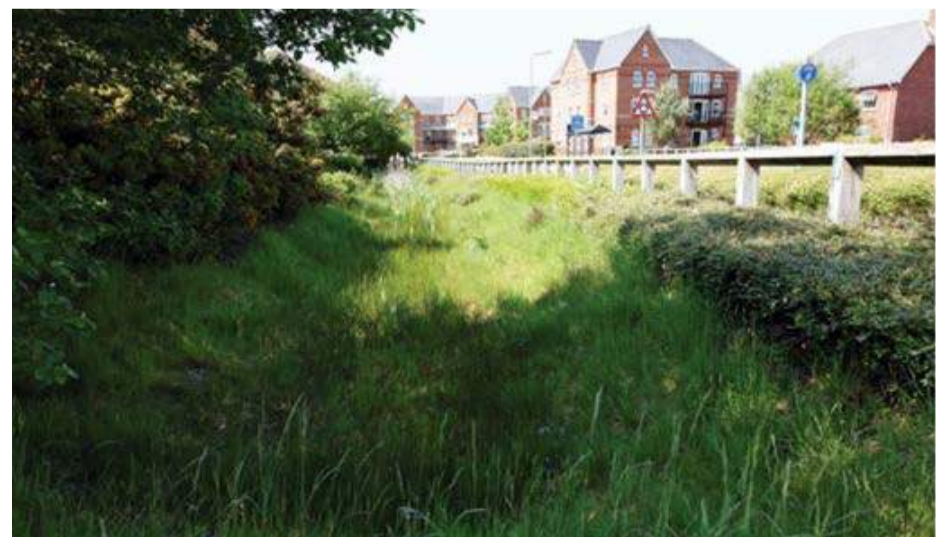
Roadside Swale, Elvetham Heath, East Hampshire
